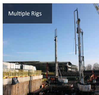
Secant Piled Retaining Wall
